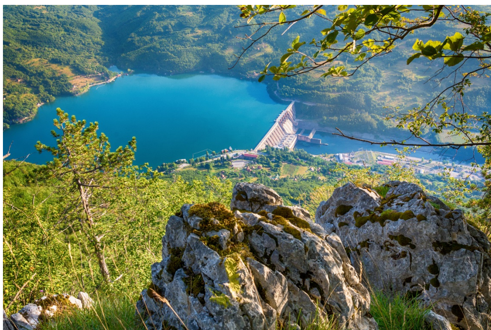
Perucac Hydropower Plant on the Drina.
